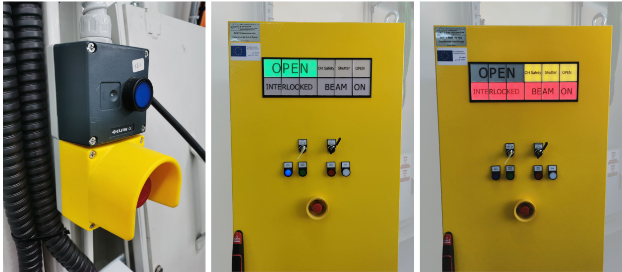
Fig. 4: (Left) PSS hutch search button. (Center) PSS cabinet; hutch is ready to start search. (Right) PSS showing hutch door interlock and beamline shutters OPEN.
